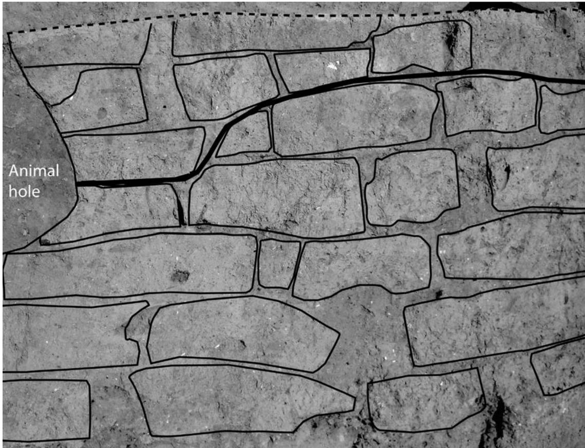
Fig. 1. A section drawing of a wall at Tell el-'Adliyyeh in Jordan, showing two building phases divided by a thick black line. The lower wall was restored after a period of abandonment with new mud bricks. Courtesy L. P. Petit.
